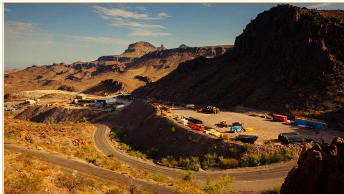
Shop facility and laydown
