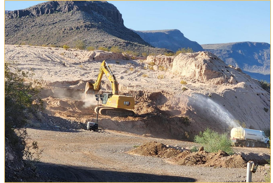
Excavator at the Reed tailings site
